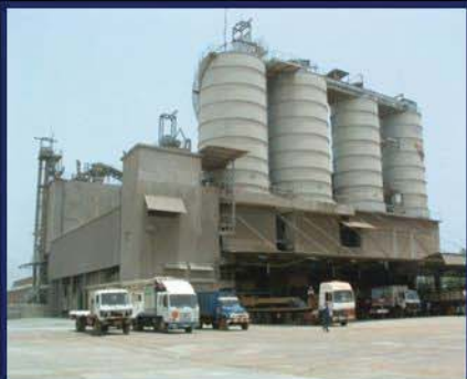
Project: Rehabilitation and Reconstruction of Cimtogo Role: Design / Build Client: Cimtogo – Lome, TOGO
