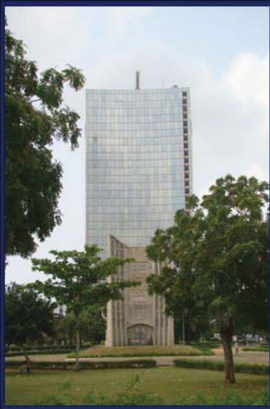
Project: Full Rehabilitation and Reconstruction of the tallest building in Togo Role: Design / Build Client: LAICO – from Libya
